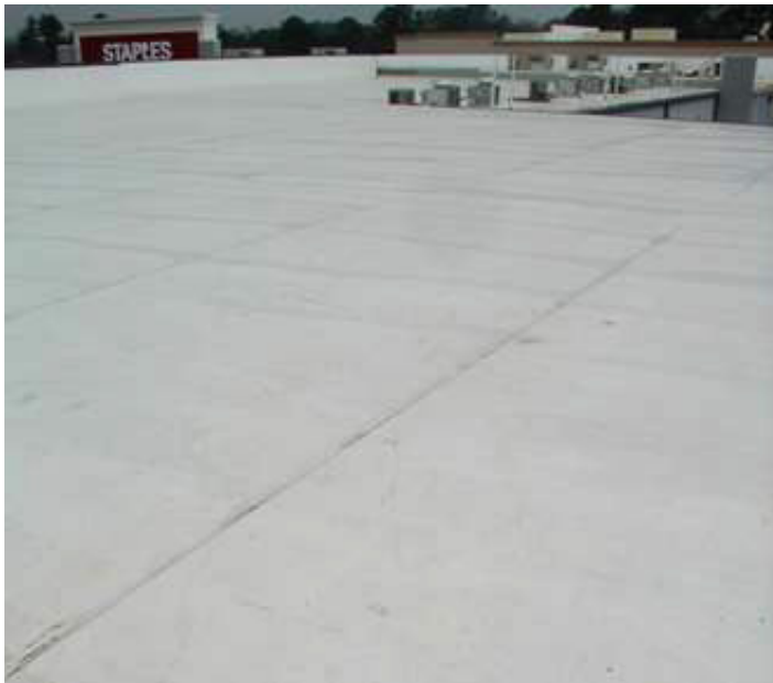
Example of a TPO roof system
